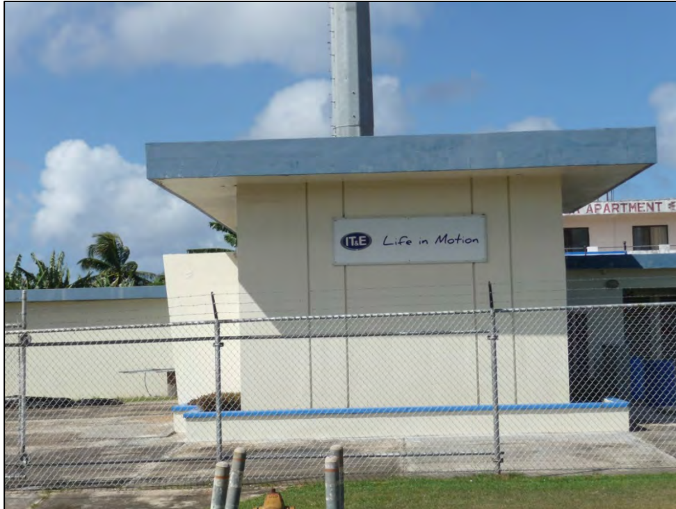
Photo 2.1-1. Existing IT&E Cable Landing Facility on Tinian
